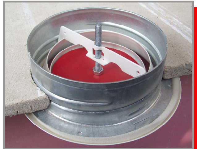
MANROSE Fire Air Valve installed before a fire
